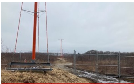
8 New Fence at North Central State Airport
