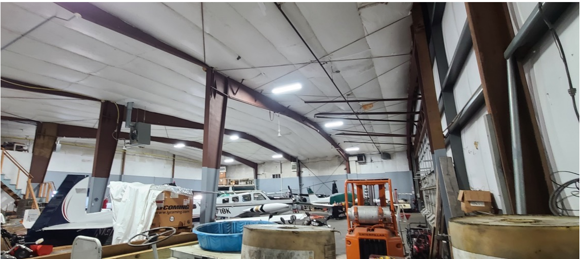
Conditions in Newport State Airport Hangar before construction
