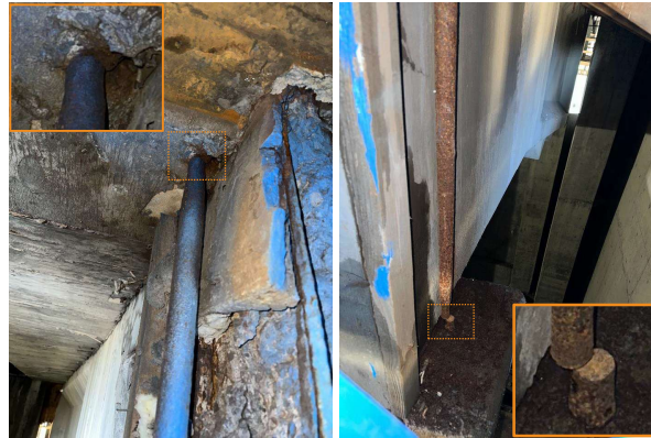
Figure 2. Pier 7 Cantilever A fractured tie-down rod
