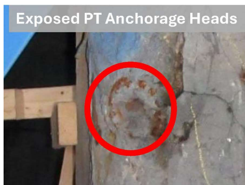
Exposed PT Bearing Plate
