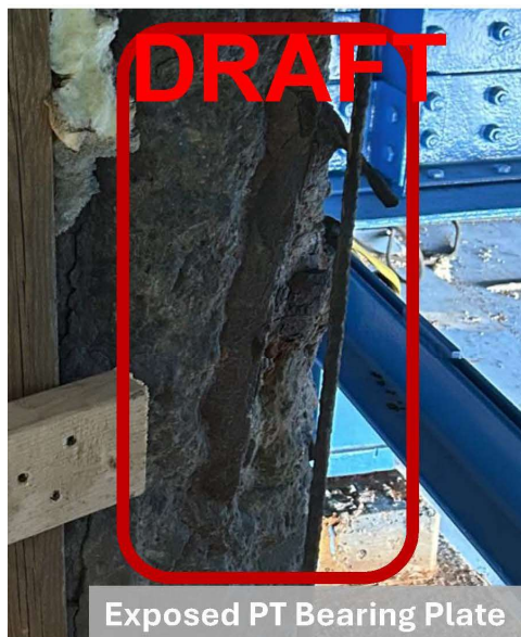
Exposed PT Anchorage Heads
