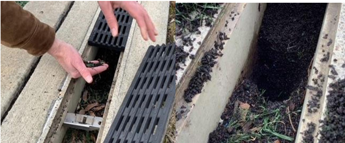
Tire-waste crumb rubber infill and broken plastic blades in artificial turf field perimeter drain (Arlington, MA 2022)
