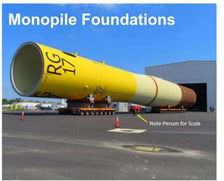
"Giant hammers ram the turbine's upright steel tube called a monopile that weighs 2,000 tons, into the seabed" --GE Turbine Website
